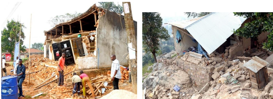
Figure 3.2: Brick Masonry (left) and adobe mud block (right) building which suffered complete damage during the 2016 earthquake (AFP 2011).
